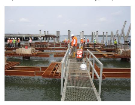
Step 3: Installation of reinforcement and casting concrete of transverse and longitudinal beam
