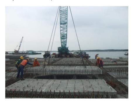
• Step 5: Installation of reinforcement and casting of topping concrete
