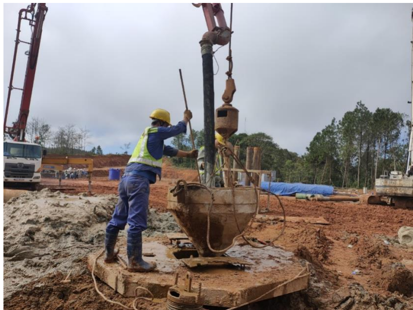
Step 1.4: Casting concrete of bored pile
