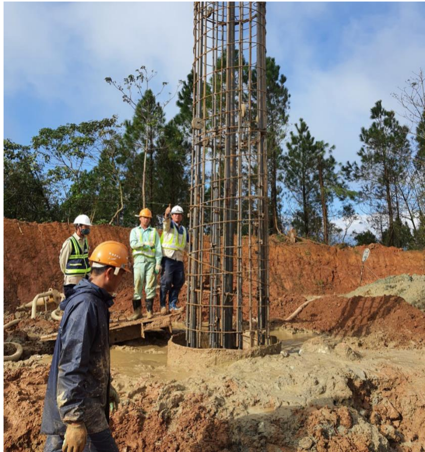
Step 1.4: Casting concrete of bored pile
