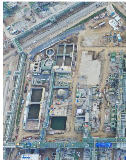
PETROCHEMICAL COMPLEX IN SOUTH OF VIETNAM
