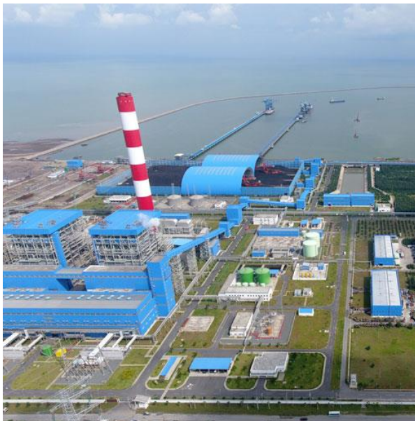
DH2 THERMAL POWER PLANT
